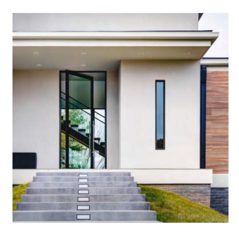
The unique weight distribution of pivot doors means they are easy to operate – even when they are oversized in height or width.
